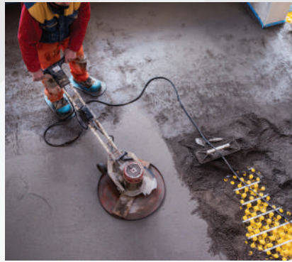
Water tanks and screed
