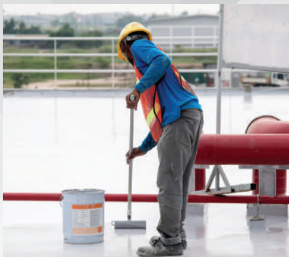
Waterproofing roof slabs
