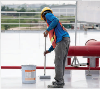
Waterproofing roof slabs
