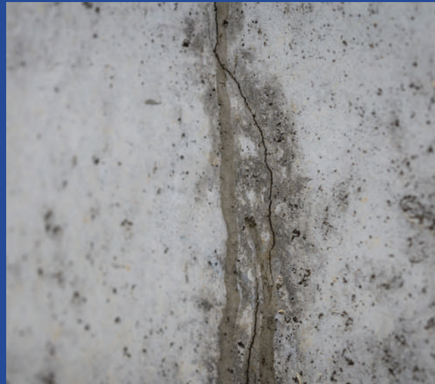
For stoppage of water inflows from cracks, joints, etc.
