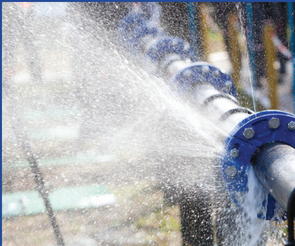
Sealing of burst pipes
