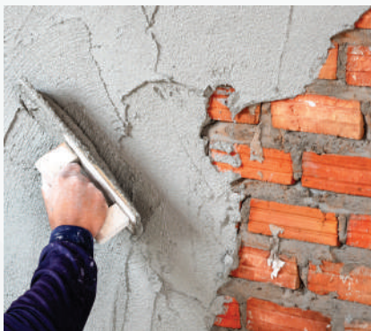
Plaster over brick masonry
