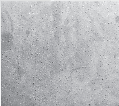
As a preventive waterproofing
